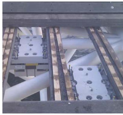
Installation under bridge
